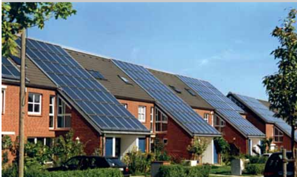
Solar Village Hamburg-Bramfeld (first big solar village in Germany)
