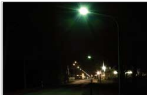
The old equipment, fitted with two 125W mercury-vapor, high-pressure discharge lamps, can be seen in the foreground.
